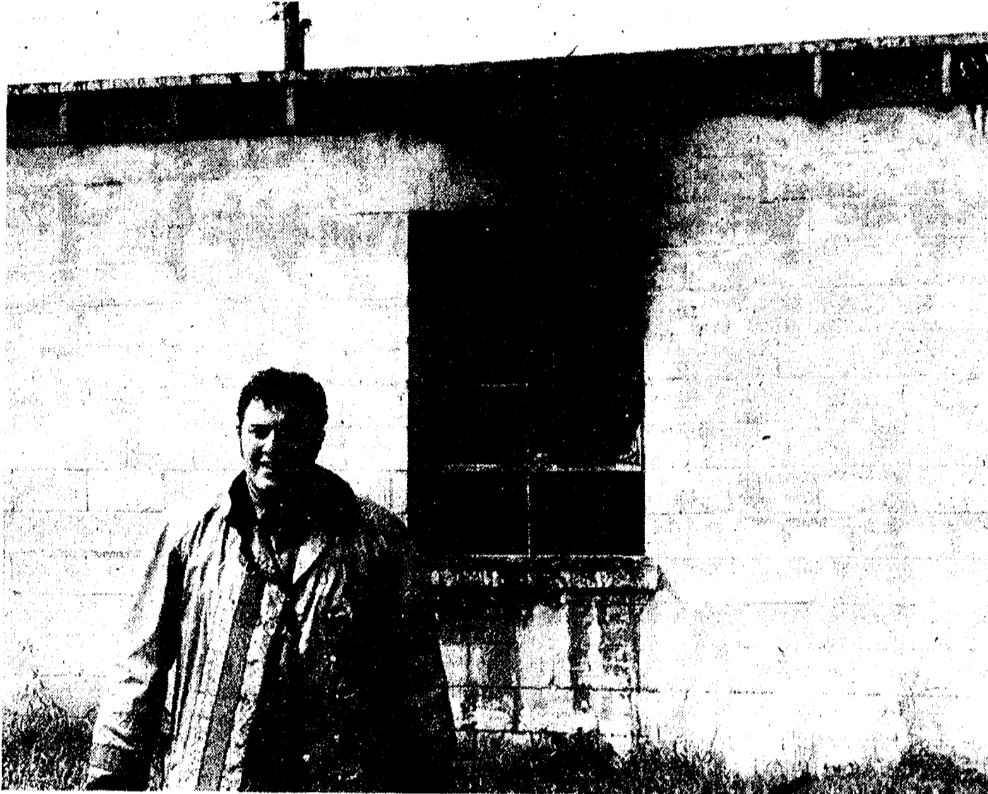
CHELSEA FIREFIGHTER Larry Gaken stands before a water drenched Central Fibre storage building shortly after firemen succeeded in dousing a blaze there last Wednesday about 3:30 p.m. The department speculates that the
